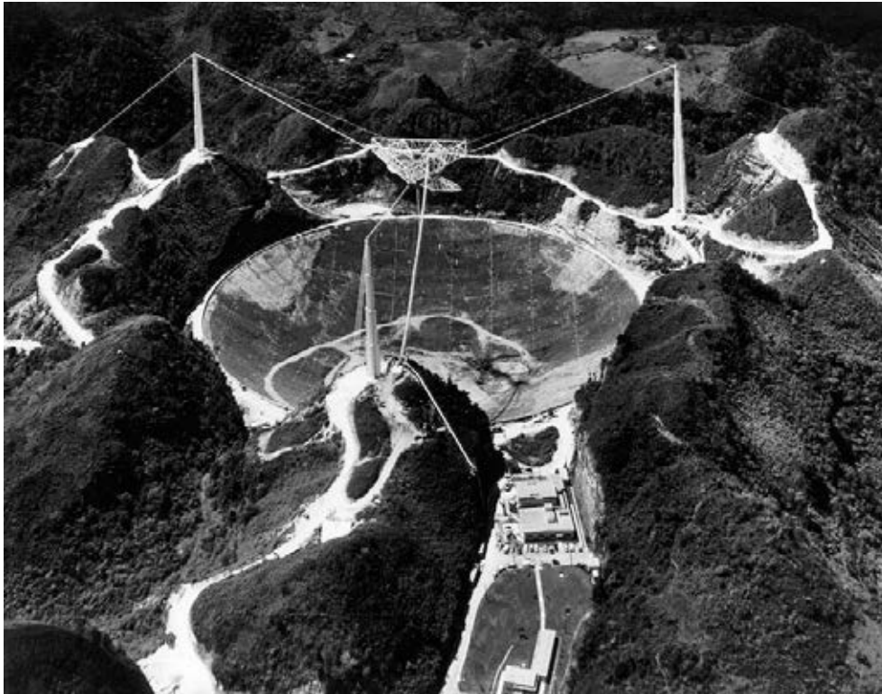
Figure 3. AIO at about the time it was dedicated on 1 November 1963. Note the 430 MHz linefeed projecting below the elevation arm – see Fig. 5 for a close-up picture of this linefeed. The waveguide from the transmitter located in the left side of the building nearest the dish is mounted above the catwalk that reaches from the triangle to near the base of the tower nearest the buildings and is then seen to reach from this point to the top of the cliff above the transmitter/operations building. Photo courtesy of Cornell University and Arecibo Observatory.
