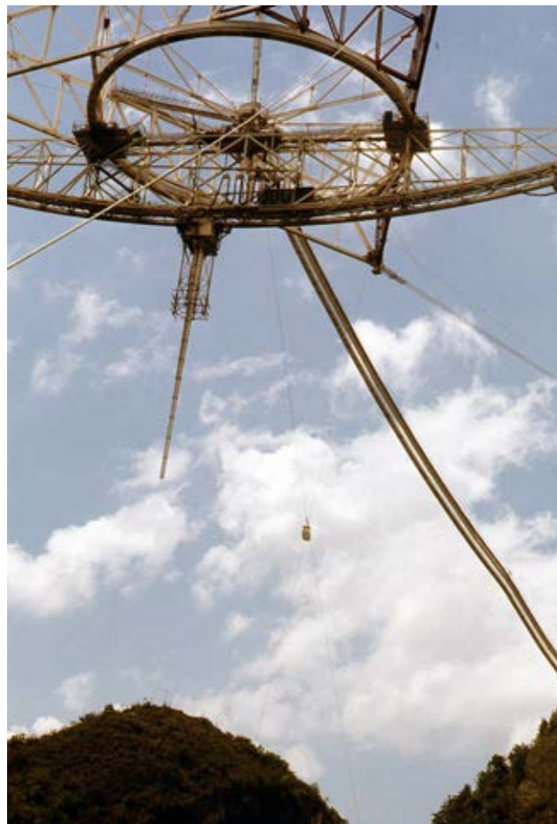
Figure 5. A picture from 13 May 1971 showing carriage house 1 (CH1) with the 40 MHz radar feed system consisting of four Yagi antennas placed symmetrically around the original square cross-section 430 MHz linefeed. Note the cable car giving convenient access to the platform relative to the catwalk which is located to the right and above the cable car in this photo. Photo courtesy of Cornell University and Arecibo Observatory.
