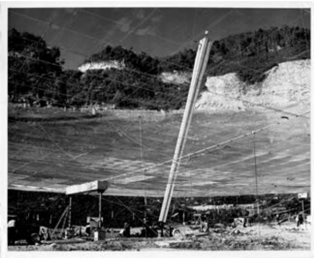
Figure 2. The original 430 MHz square cross-section linefeed as it was raised to the carriage house in this photo dated 14 August 1963. Photo courtesy of Cornell University and Arecibo Observatory.
