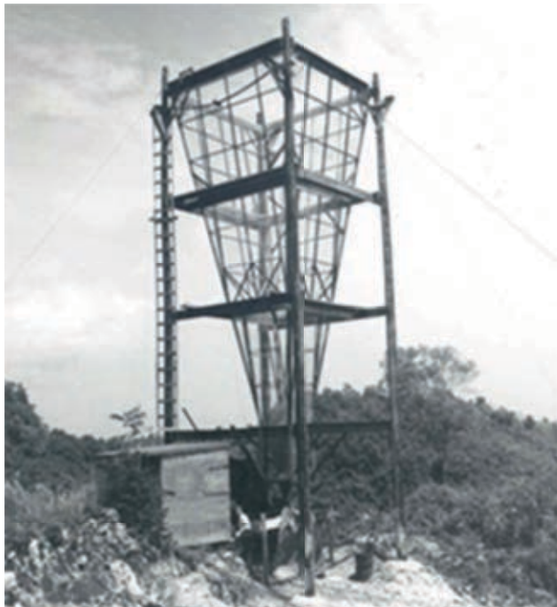
Figure 4. The first functioning radar feed at AIO. This 430 MHz hornfeed was constructed to test the full radar system before the dish was completed. This feed had a \sim 10^\circ half-power beamwidth and was in operation in mid-October 1962. It was used to receive the sun in transit and to obtain lunar echoes as the moon transited near zenith (Gordon, 1962a). Photo courtesy of Carmen G. Segarra-Saavedra (Segarra-Saavedra, 2012).
