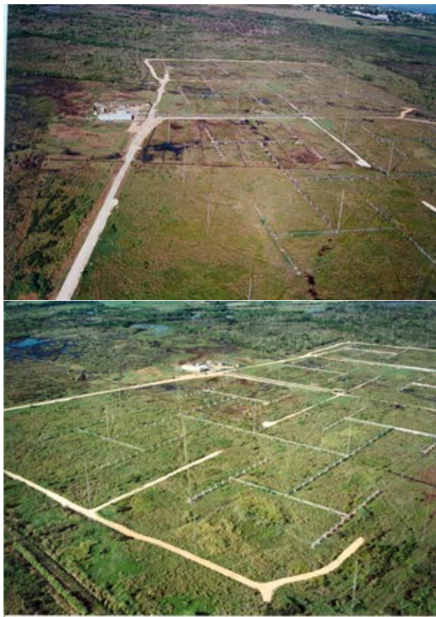
Figure 7. The Islote heater facility circa 1997. In these aerial views most of the two 4 \times 4 log periodic antenna arrays is visible with the transmitter/control building to the left/top and the ocean just visible at the top right. The dual, closed coaxial “cable” (constructed from irrigation pipe) transmission line system to the center of each log periodic feed is clearly visible as are the support towers. The wire log periodic feeds are not visible but are suspended from four towers with two linear polarizations each driven from a separate transmission line. Photo courtesy of Cornell University and Arecibo Observatory.
