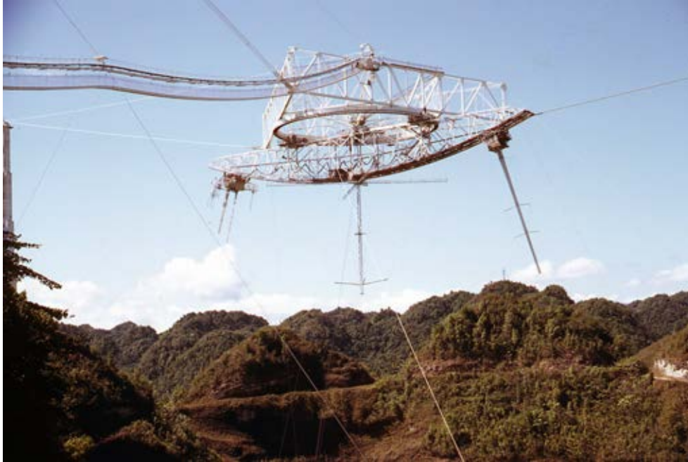
Figure 6. The Arecibo Observatory feeds in July 1972. The new 430 MHz linefeed is mounted on carriage house #1 to the right in this photo. In the center is the HF log-periodic feed for ionospheric heating experiments. To the left is carriage house #2 with various radio astronomy feeds including those at 318 MHz (left, 40 feet long), 611 MHz (right, 45 feet long), the far-right feed is likely 1667 MHz test feed while the feeds at the far left are likely nested Yagis at 111 MHz and 196 MHz (D. B. Campbell, personal communication, 2013). Note the catwalk at the upper left of the photo. Photo courtesy of Cornell University and Arecibo Observatory.
